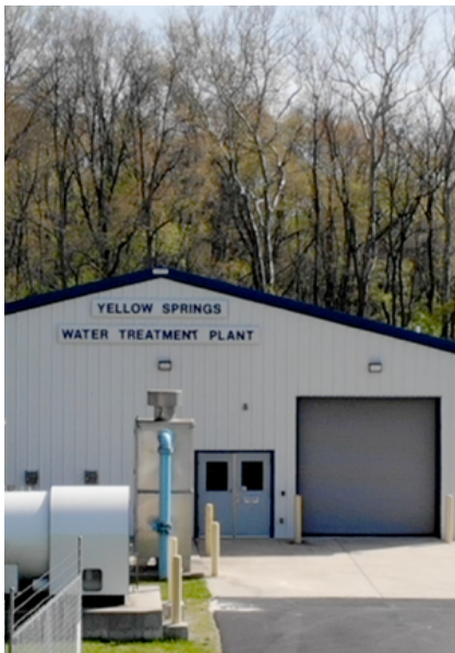
Yellow Springs Water Treatment Plant
