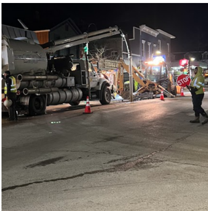
Water main break repair on Xenia Avenue
